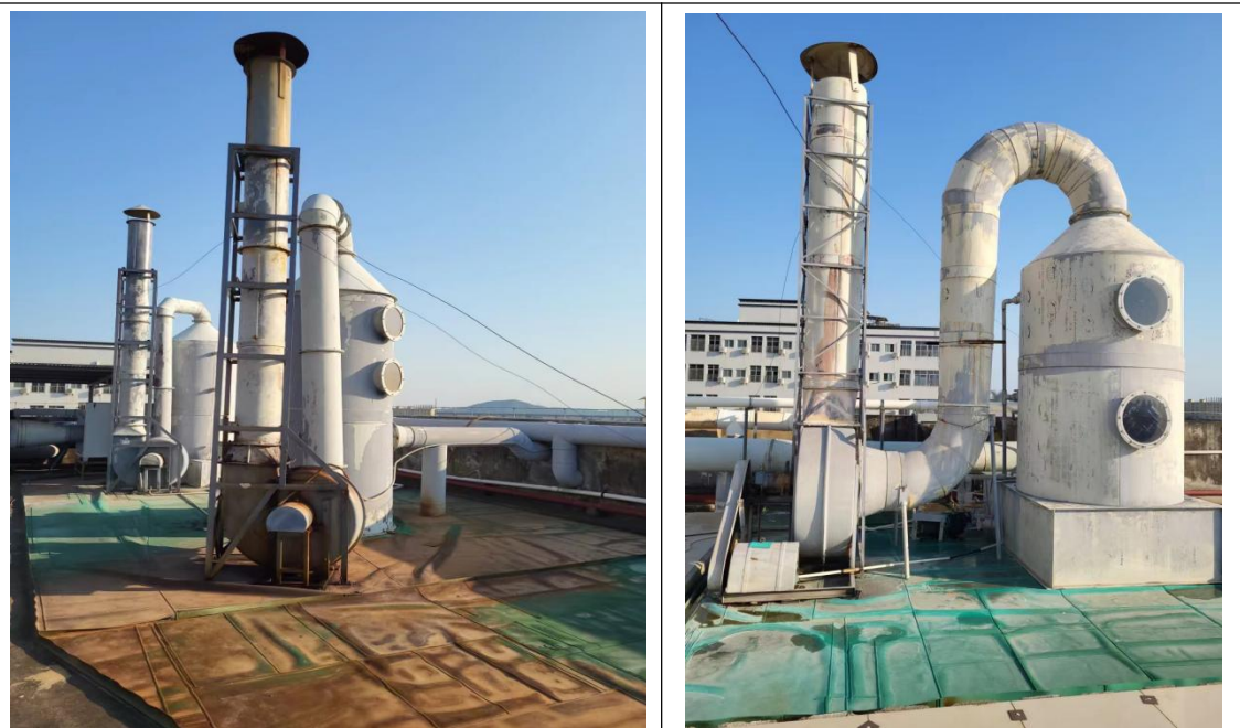
酸雾废气碱喷淋设施
